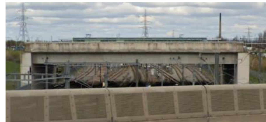
Podium UK example. High Speed 1 Ebbsfleet, Kent, 50m*50m to accommodate potential future development
