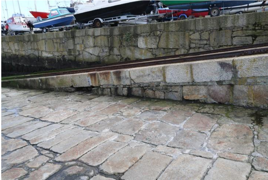
Plate 11: Western side of the lower part of the western ramp
