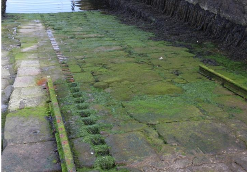
Plate 53: View down the lower part of the patent slip
