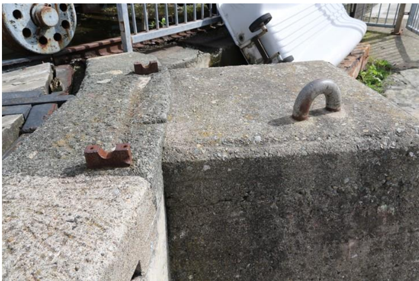
Plate 46: Bearings and ring on south-western side of turntable.
