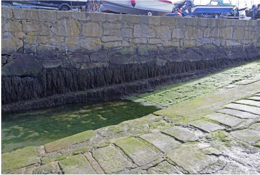
Plate 7: Lower end of patent slip, seen from main slipway
