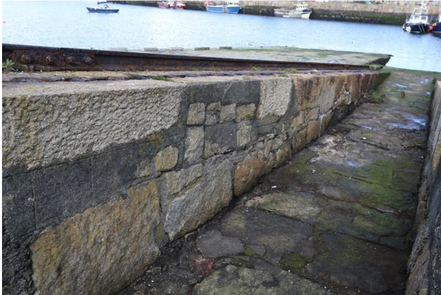
Plate 13: Eastern face of western ramp at lower level
