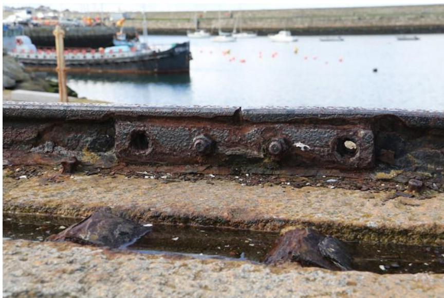
Plate 50: Fishplate joining rails
