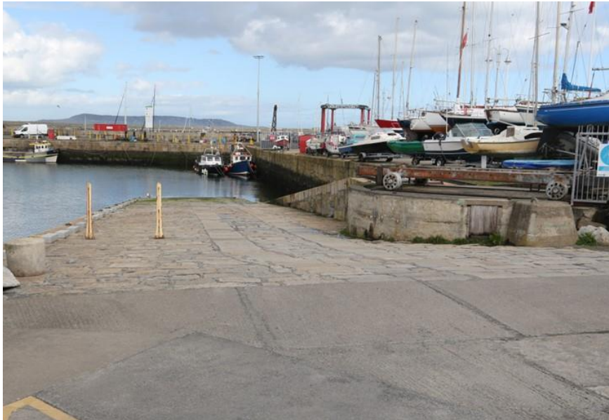
Plate 1: View of slip from landward side, looking north, with patent slip at right
