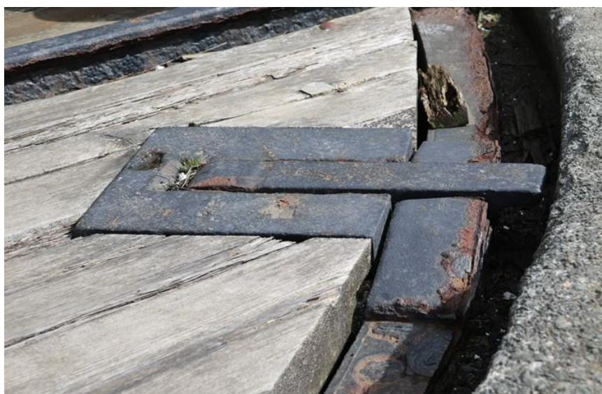
Plate 42: Lock at perimeter of the turntable
