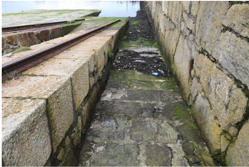
Plate 31: Area between the eastern ramps and the quay wall
