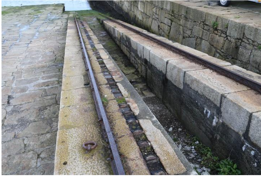
Plate 9: View down the western of the two ramps on the patent slip
