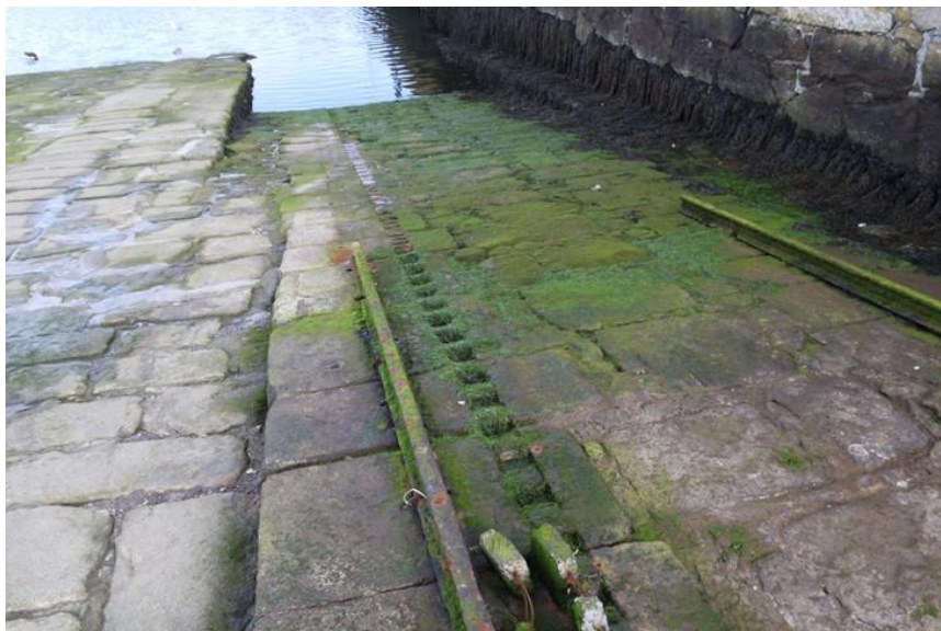
Plate 26: Area between the ramps at lower end
