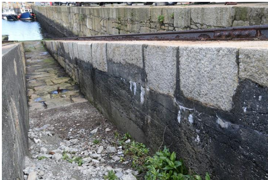
Plate 20: Western face of central section of eastern ramp
