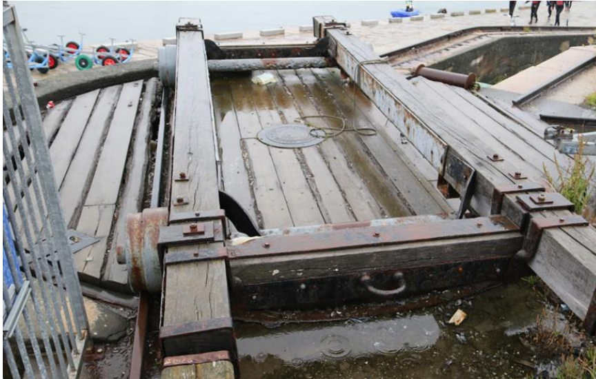
Plate 39: Boarded surface of turntable
