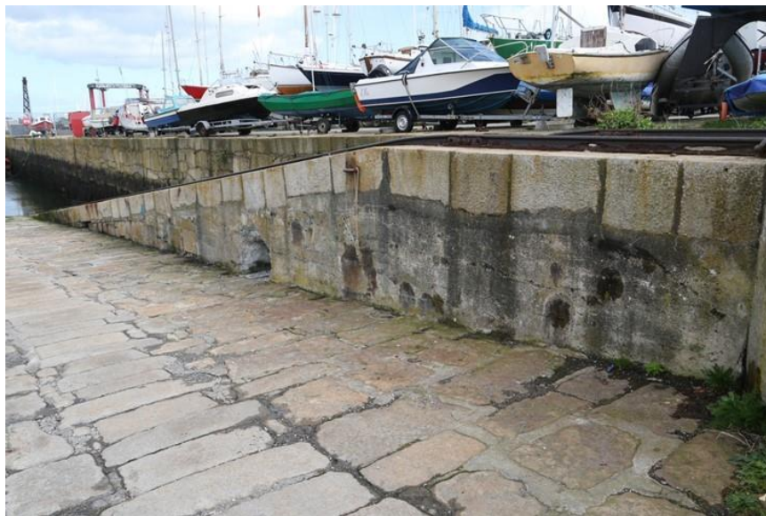
Plate 12: Upper end of the western ramp on the western side
