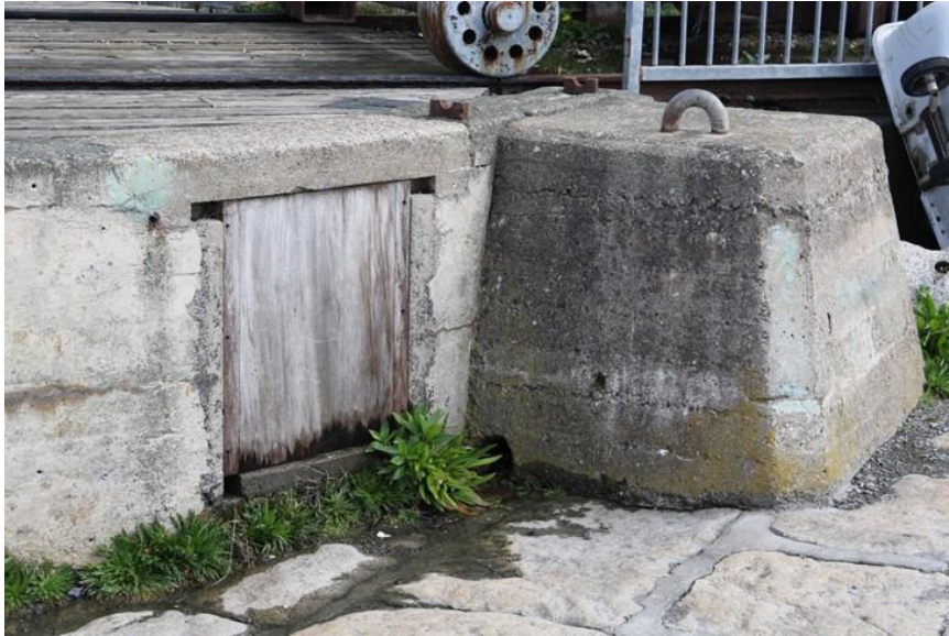
Plate 45: Door and pyramid of concrete on south-western side of turntable
