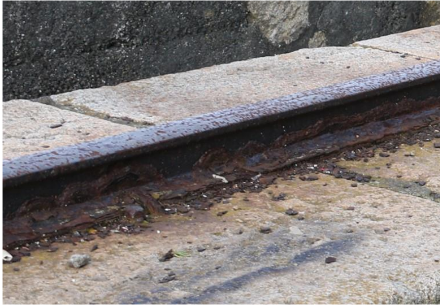
Plate 47: Detail of rail on top of ramp
