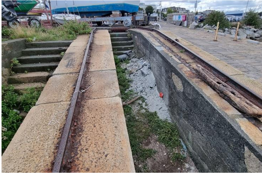
Plate 23: View to top of ramps
