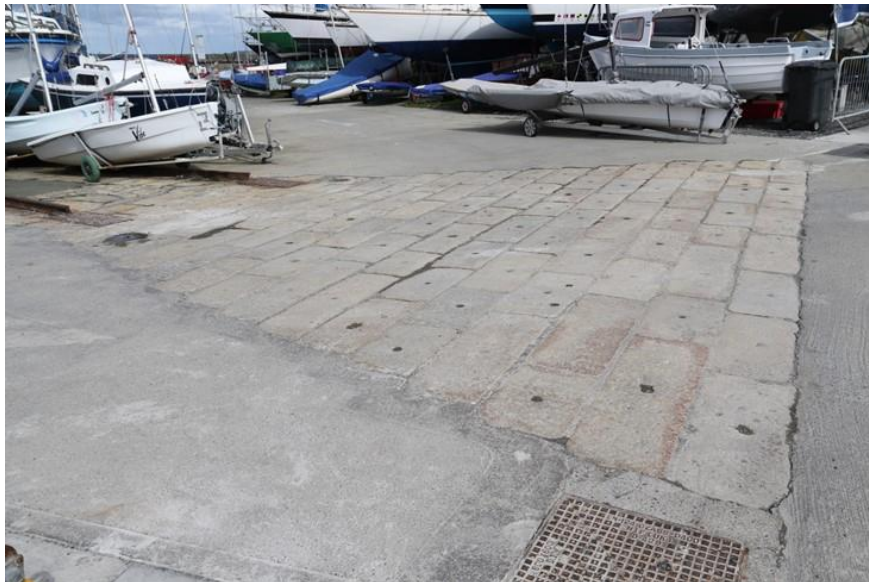
Plate 58: Paved area beyond rail siding in boatyard
