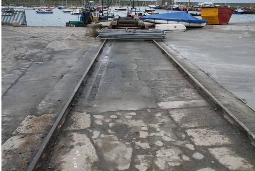
Plate 55: View toward turntable along longer rails in boatyard
