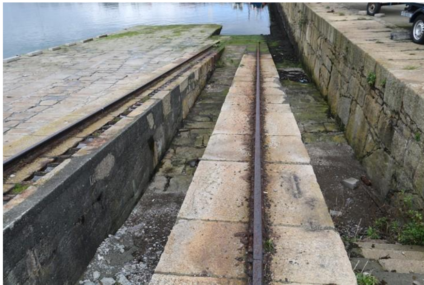
Plate 18: Middle part of eastern ramp
