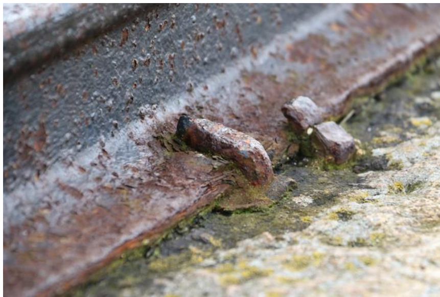
Plate 48: Detail of fixing of rail
