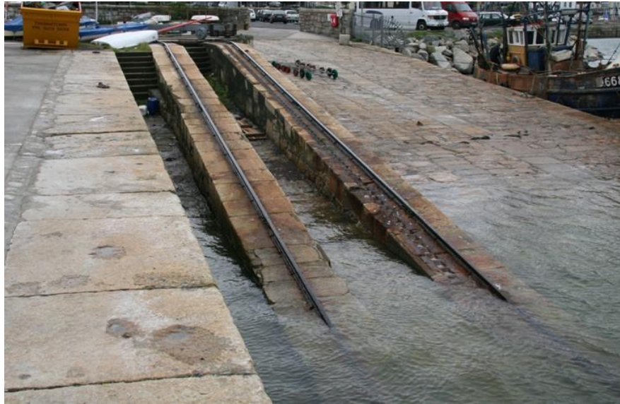
Plate 3: Patent slip, seen from the quayside at the boatyard in 2006
