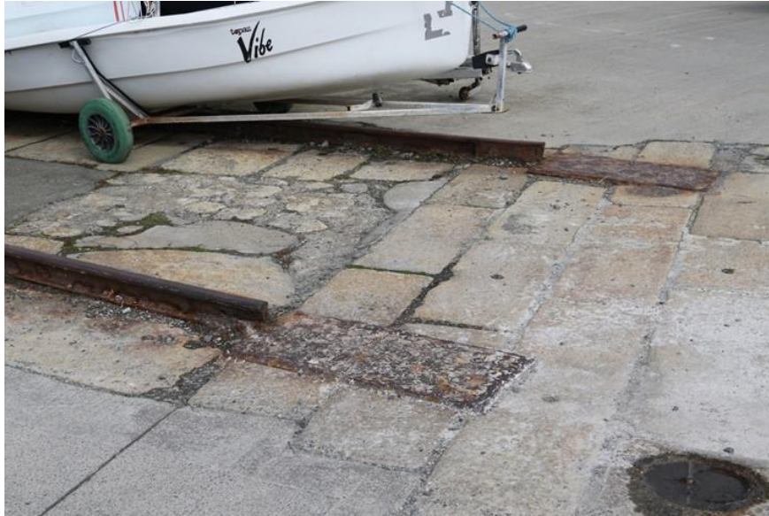
Plate 57: Southern end of rail siding at boatyard
