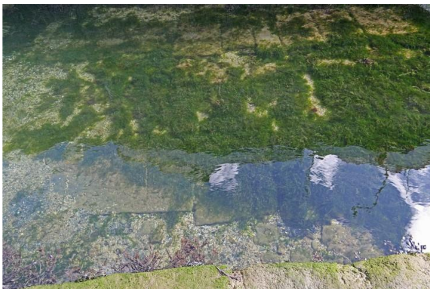
Plate 8: Lowest section of patent slip, below water level
