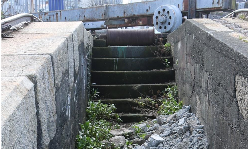
Plate 29: Steps at top of area between the ramps
