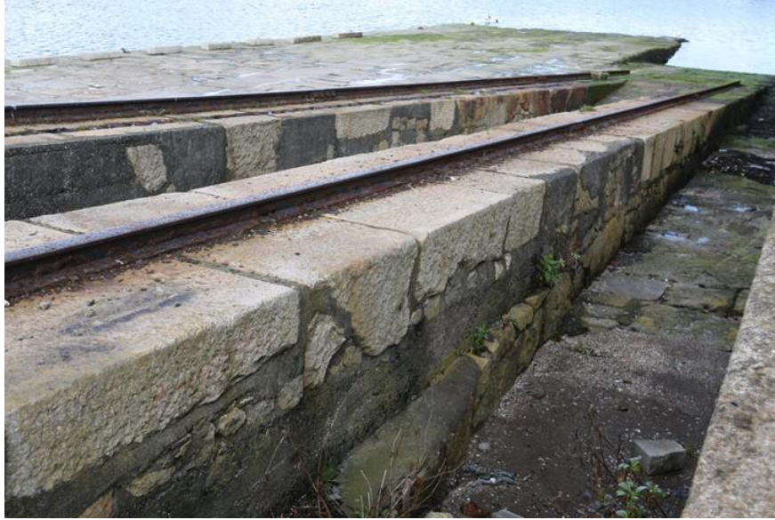
Plate 21: Lower part of eastern face of eastern ramp
