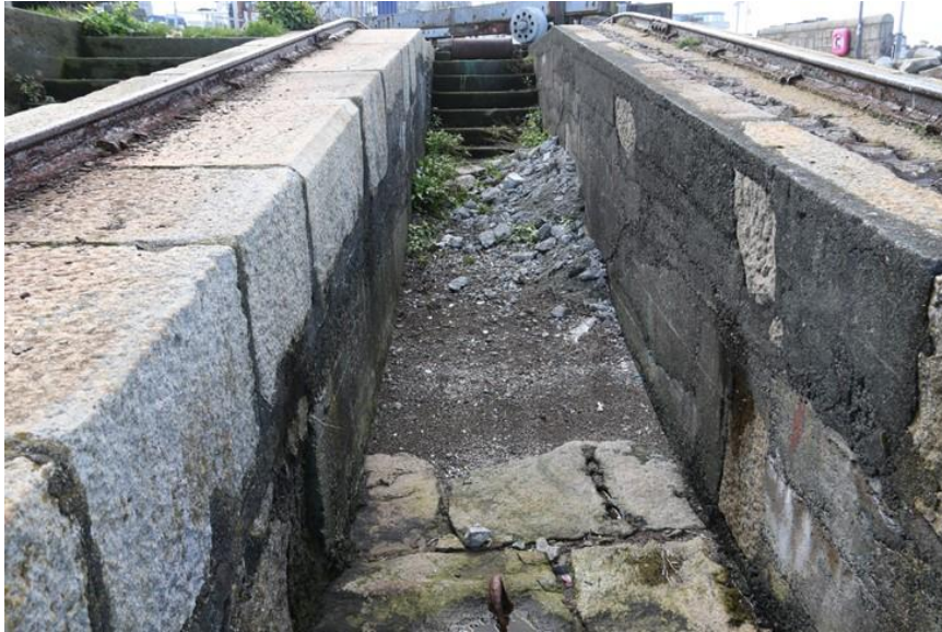
Plate 27: Upper end of area between the ramps
