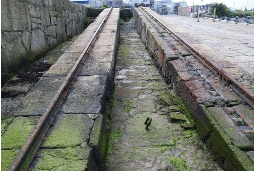
Plate 25: View between the ramps toward the top
