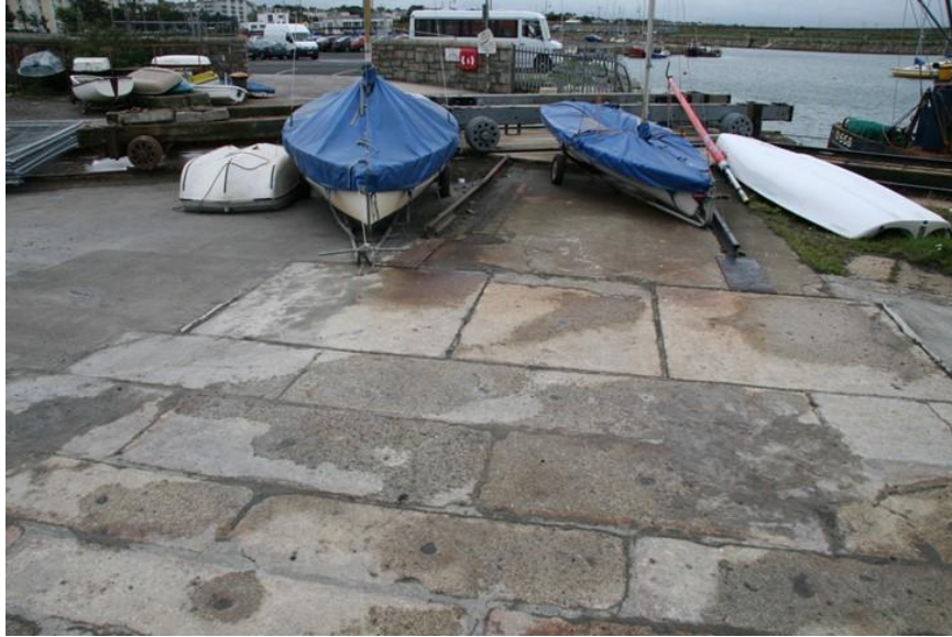
Plate 61: Paving at end of eastern siding
