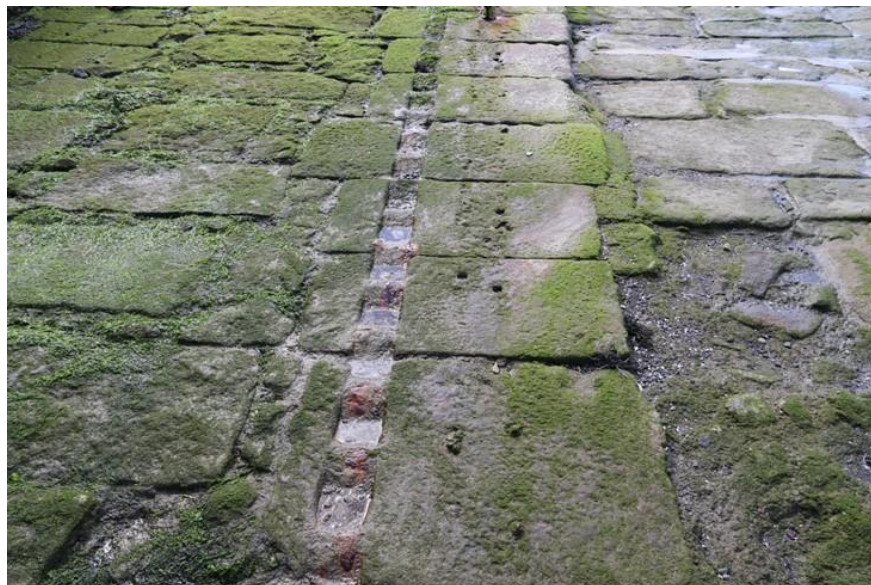
Plate 54: Detail of rack and fixings for rail on lower part of patent slip
