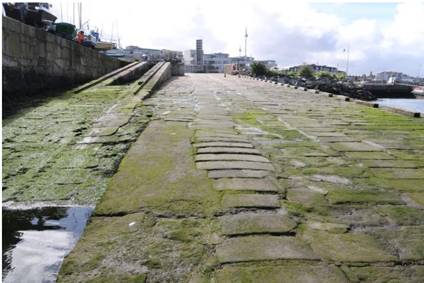
Plate 2: View up slipway with patent slip at left
