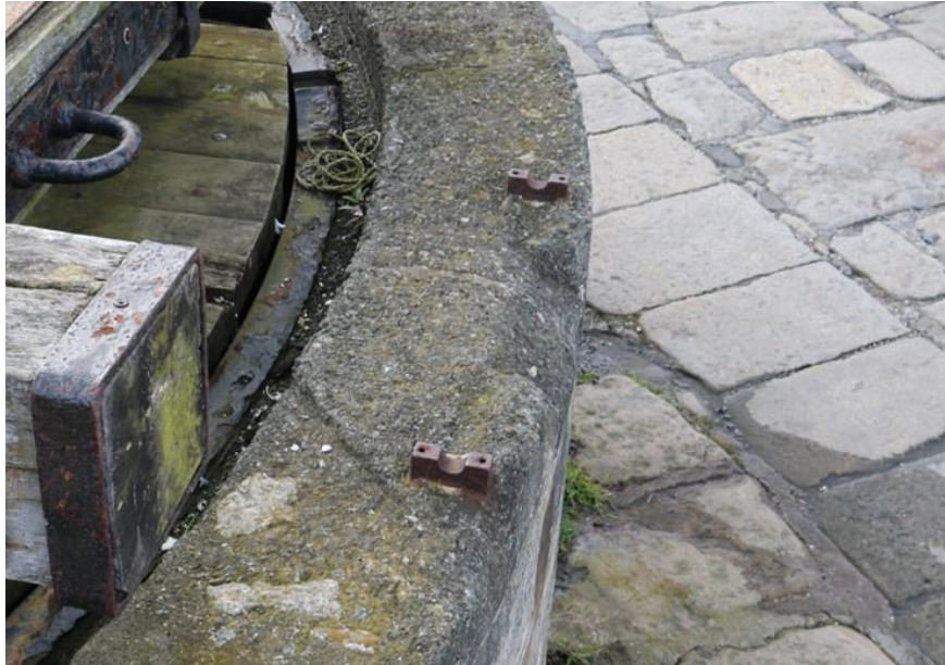
Plate 43: Seatings of bearings at western side of turntable
