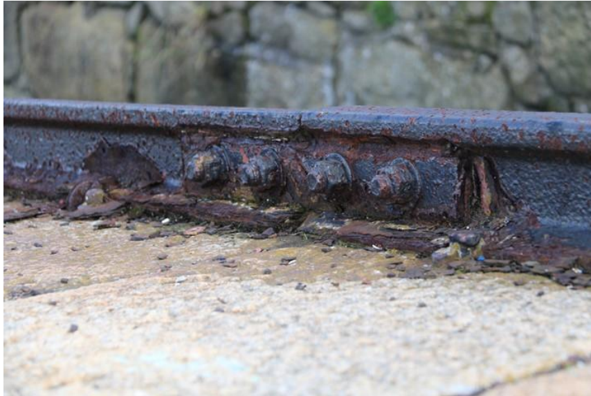
Plate 49: Fishplate joining rails
