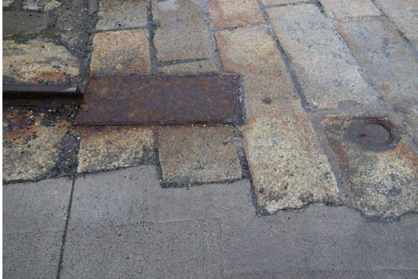
Plate 63: Plate and iron ring at end of rails on southern siding
