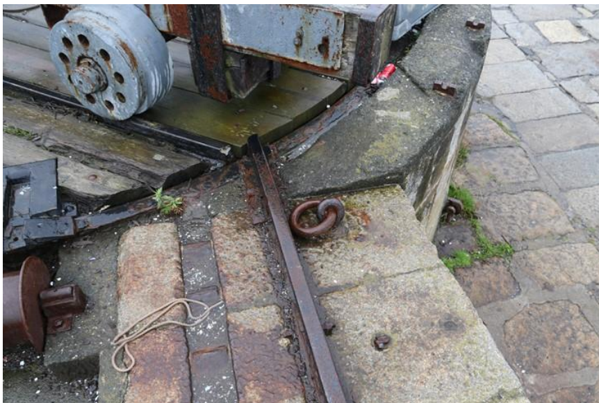
Plate 16: Iron ring at northern end of western ramp
