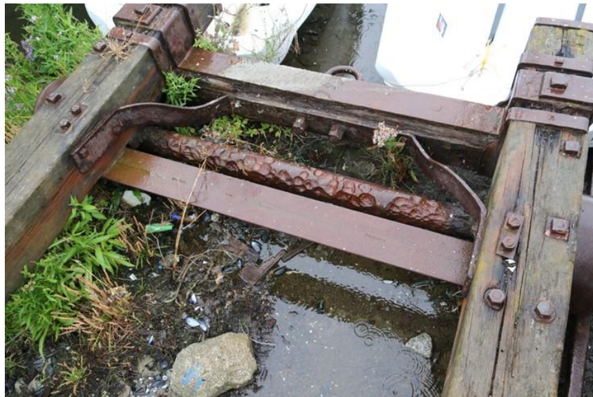
Plate 72: Detail of smaller carriage showing pitting of axle
