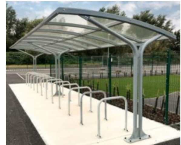
Figure 10-5: Sheltered Sheffield stands by school entrance.
