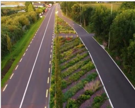
Figure 15-7 The Dunkettle to Carrigtwohill Cycleway Scheme, with SuDS in the form of a pollinator corridor. Source: Cork County Council.
