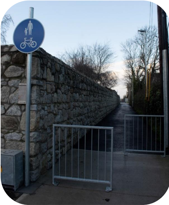
Figure 11-1: Existing filtered permeability link in Kiltiernan-Glenamuck. Source: DBFL.
