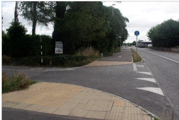
Figure 13-3: Example of a Side-Entry Treatment including a raised table on the Glounthaune Pedestrian and Cycle Scheme, Co. Cork. Source: DBFL.
