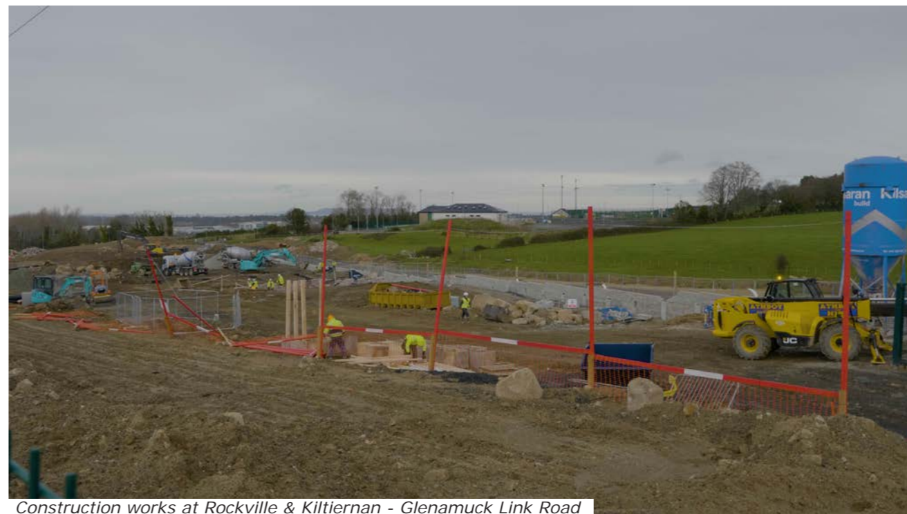
Construction works at Rockville & Kiltiernan - Glenamuck Link Road
