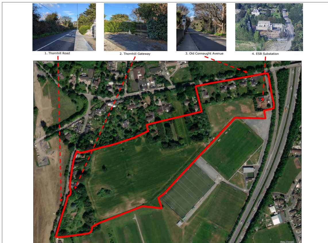
Figure 4.16: Southern Character Area on Aerial Imagery
