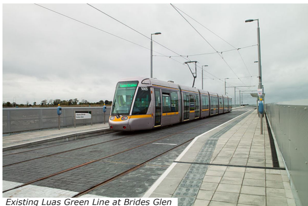
Existing Luas Green Line at Brides Glen
