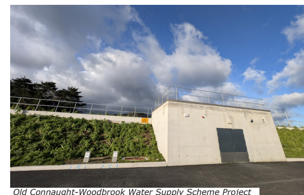
Old Connaught-Woodbrook Water Supply Scheme Project
