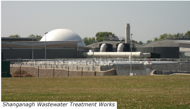
Shanganagh Wastewater Treatment Works
