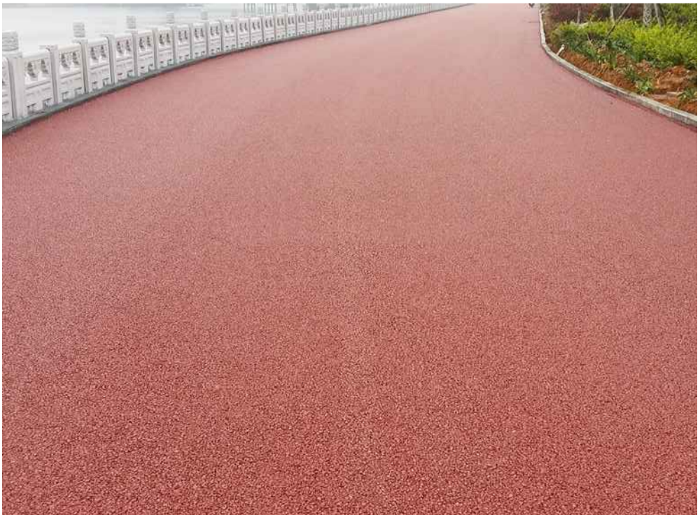
STONE MASTIC ASPHALT TO CYCLE PATH
