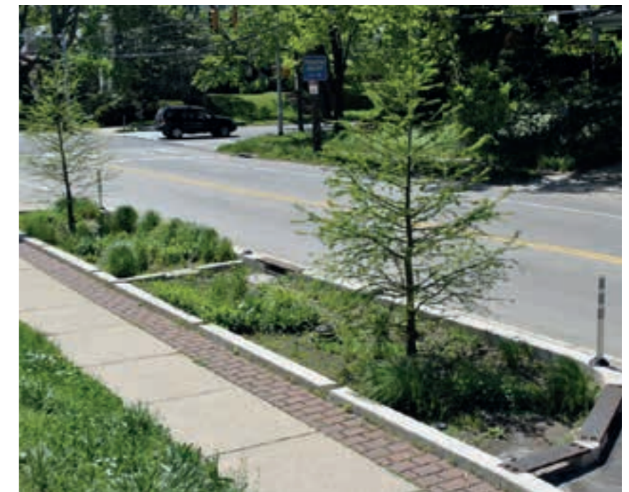
Photo 60: Stormwater Bump-Out on Queen Lane, Philadelphia. Source: Flickr. Image By: Philadelphia Water Department.
