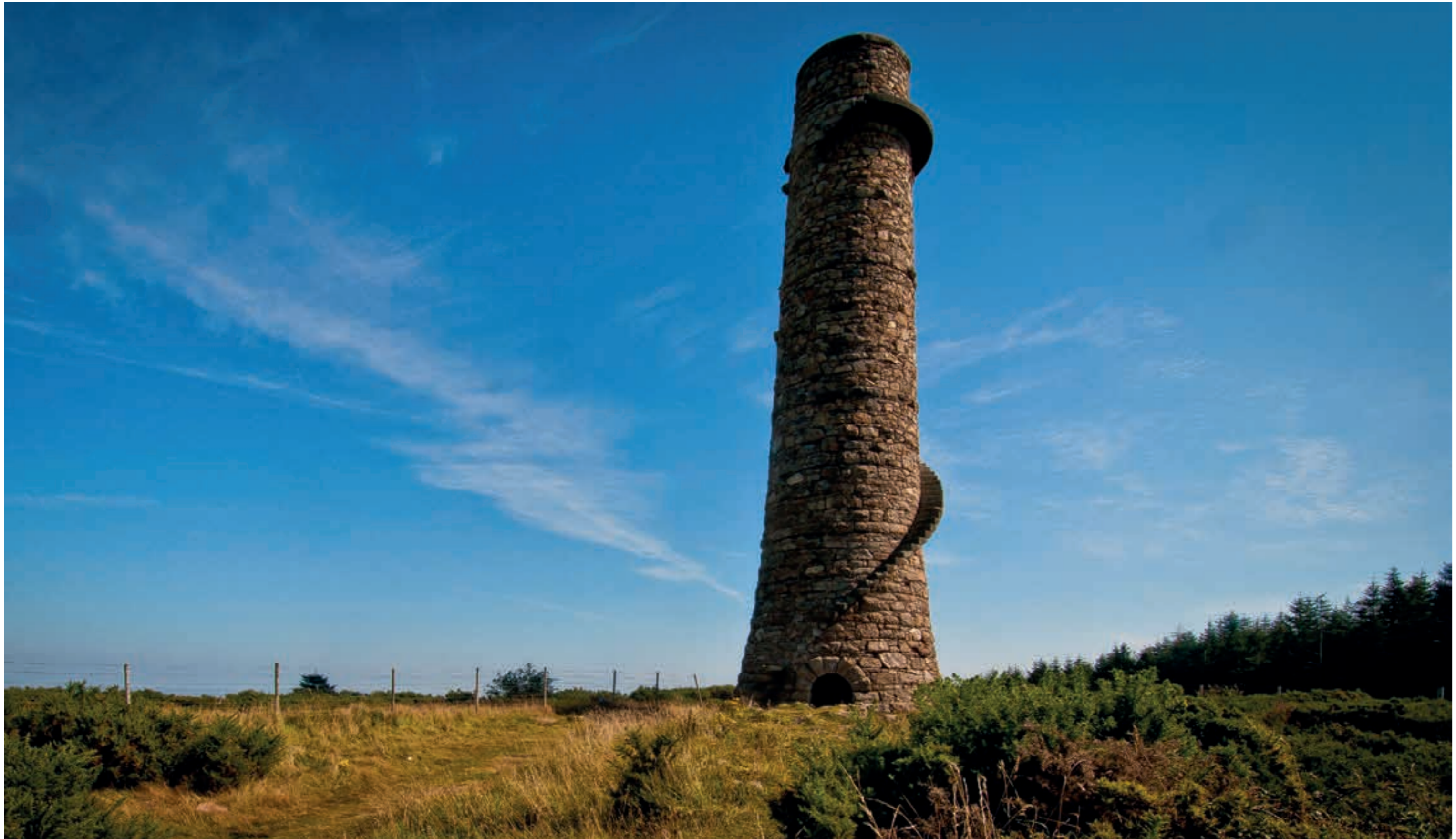
Photo 6: Chimney at Ballycorus Leadmines. Source: Wikimedia. image By: Joe King.
