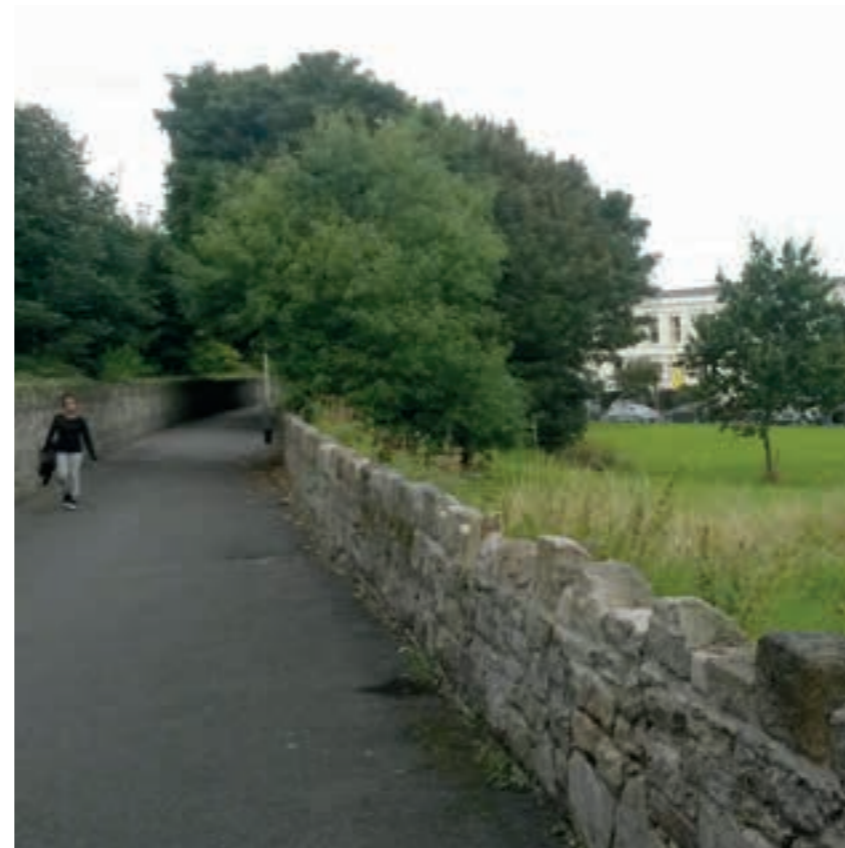
Photo 36: The Metals at Claremont Villas.
