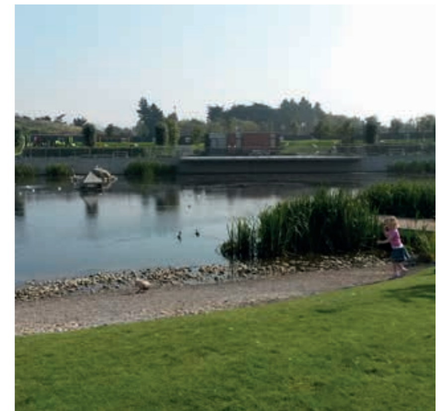
Photo 37: Attenuation Feature at Honeypark, Glenageary.
