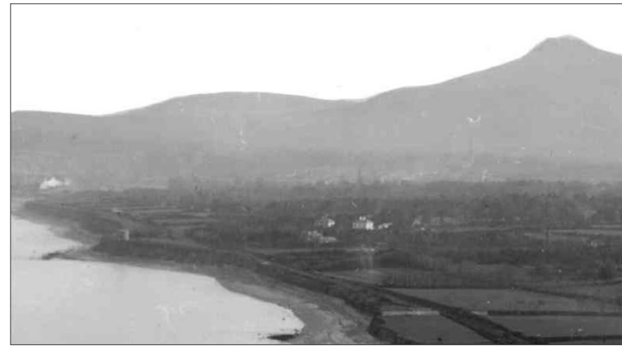
Historic aerial view of Martello Tower, 1890
